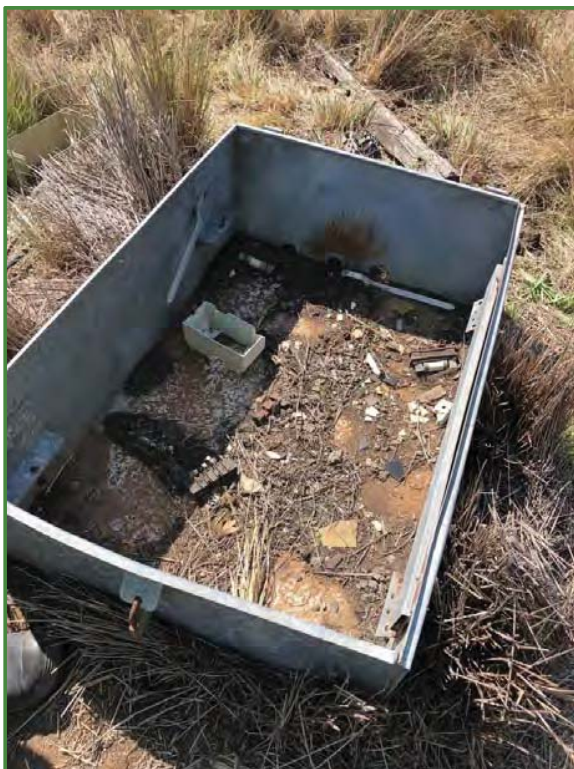
Photograph 38: Metal casing with old fuses, plastic casing and wires inside, located near the western boundary.
